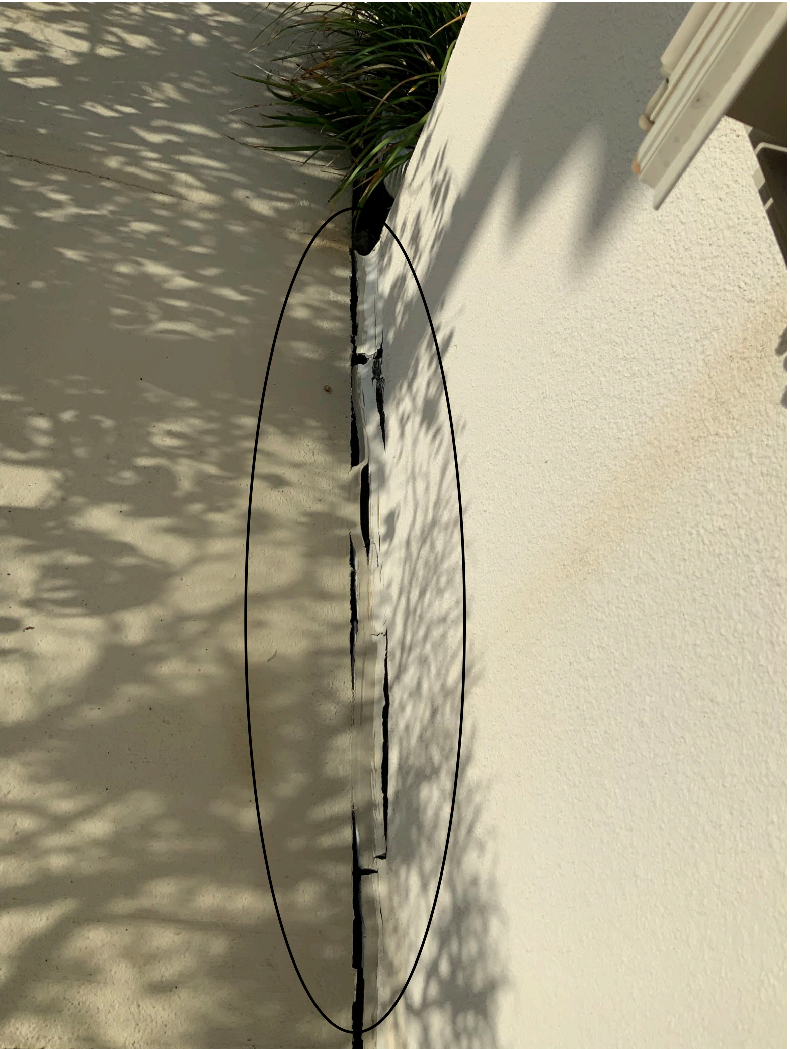
Building Separating by Sgt. Garrison's Office
